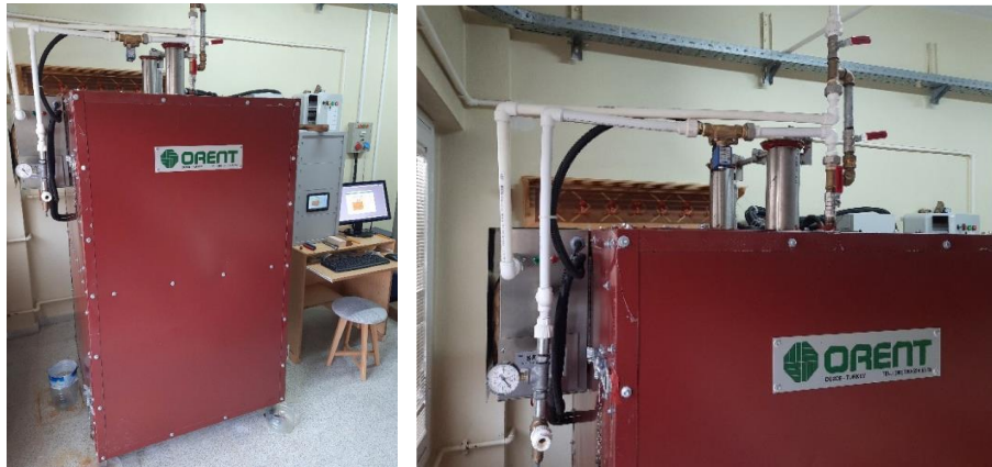
Fig. 1. Thermal treatment furnace and equipment
