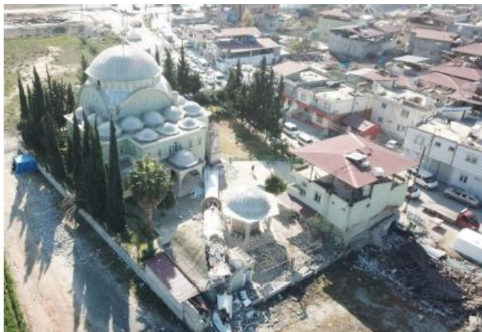
Fig. 27. Observed damages on reinforced concrete minarets
