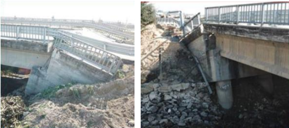
Fig. 21. Ground-foundation damages
