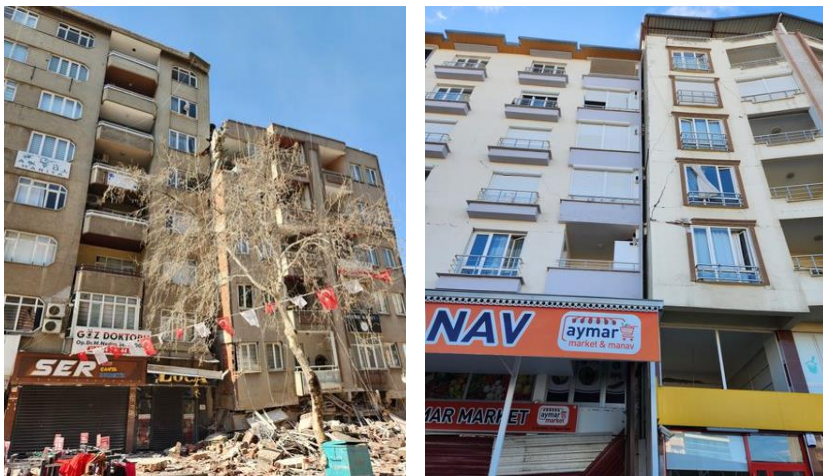
Fig. 10. Inadequate safe distance
