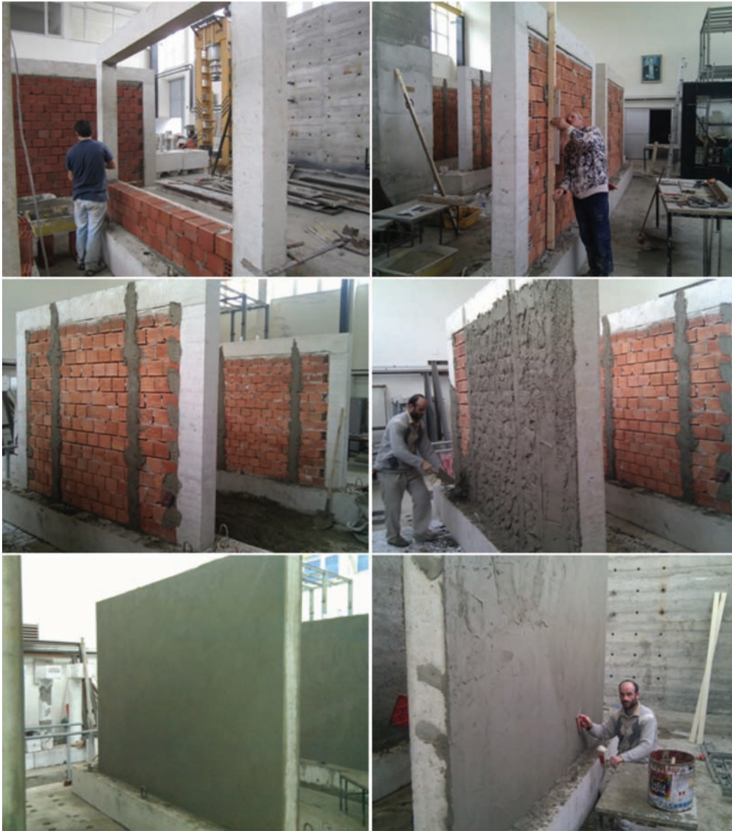
Figure 2: Application of infill wall and concrete plaster.
